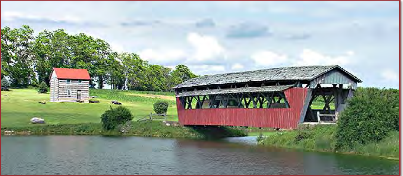
Figure 3-1: Covered Bridge Route 13 (Credit: lostbridges.org)
