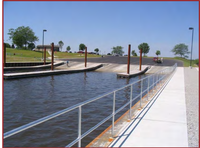
Figure 3-10: Boat Ramp (Ohio State Parks)
