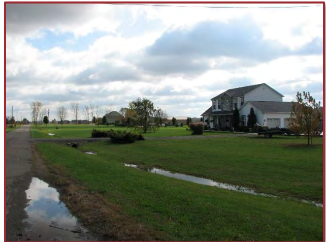
Figure 3-21: Rural road ditch and culvert
